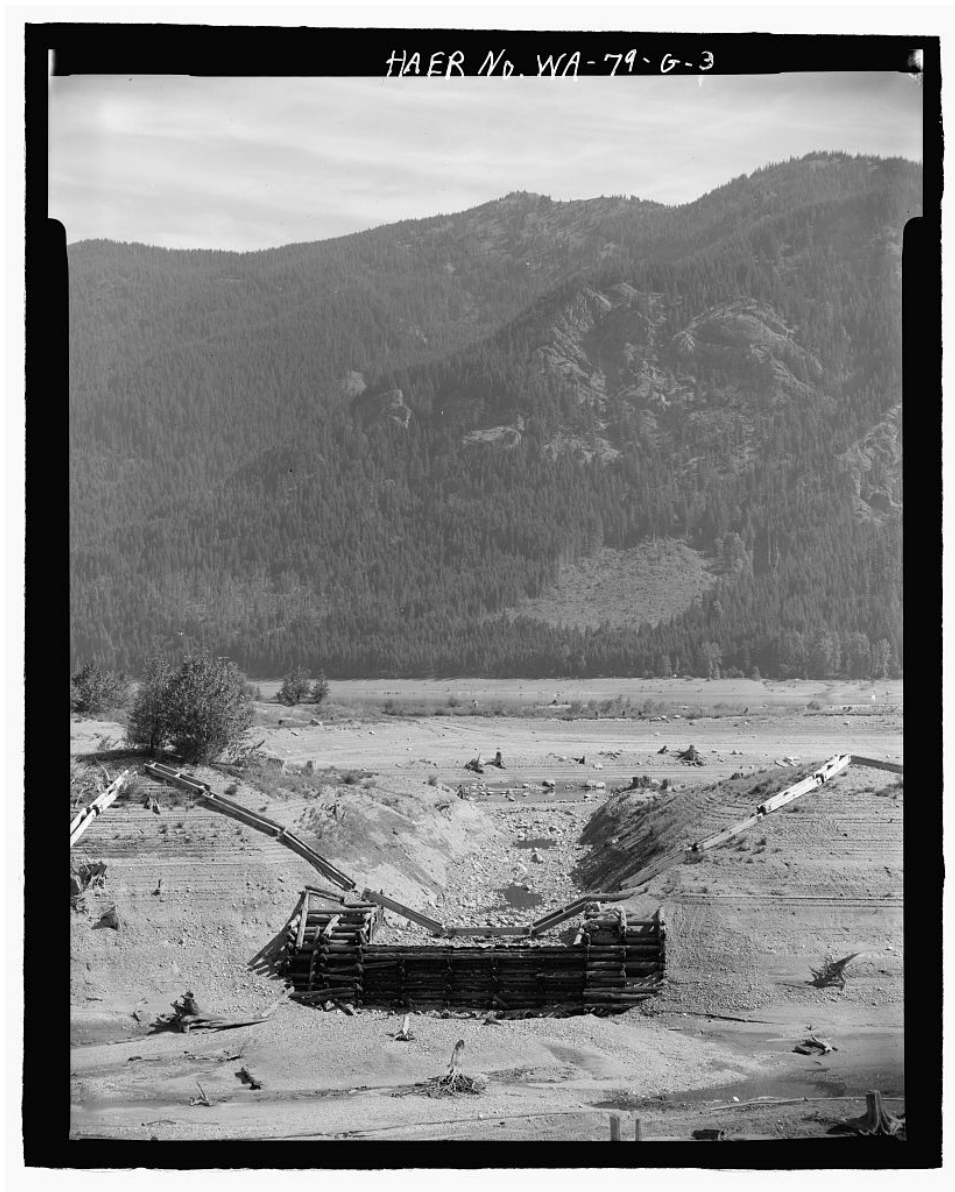
Photograph 3-6 Kachess Dam Construction 1910
